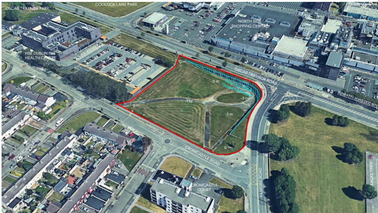
Image above: Existing Site Overview
